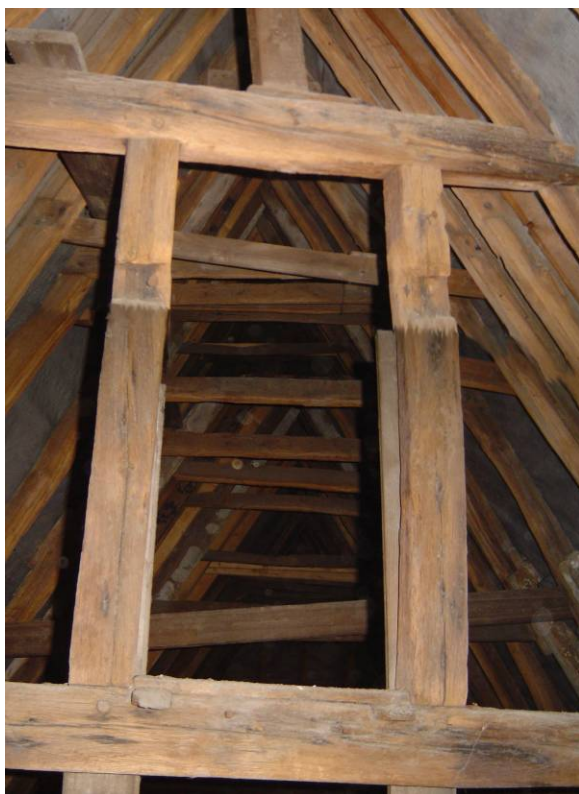
124 Raamopening in houten gevel
